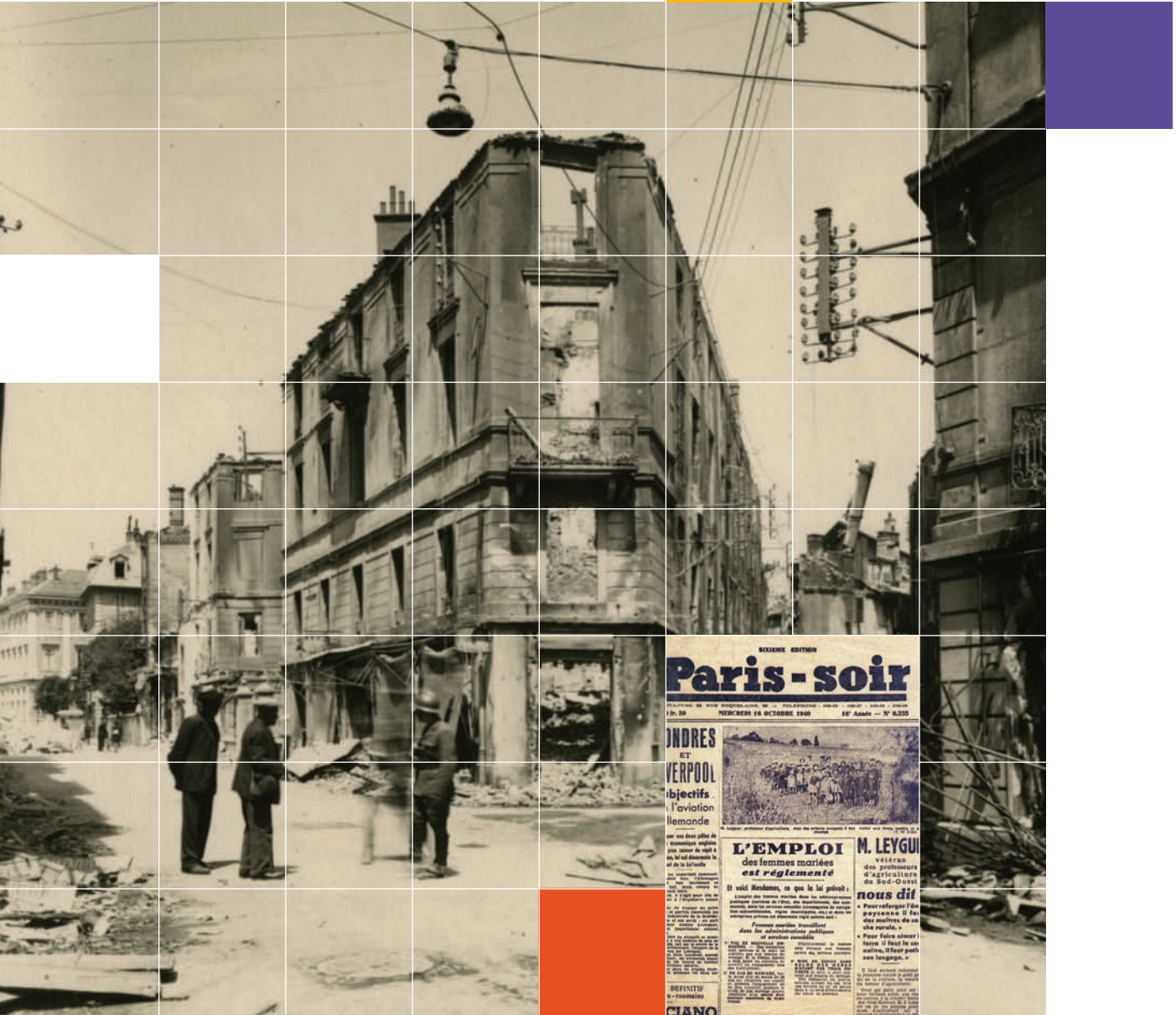
In Chambéry, the Etablissements Pillet, a subsidiary of Descours & Cabaud, suffered merciless bombing in 1944.
