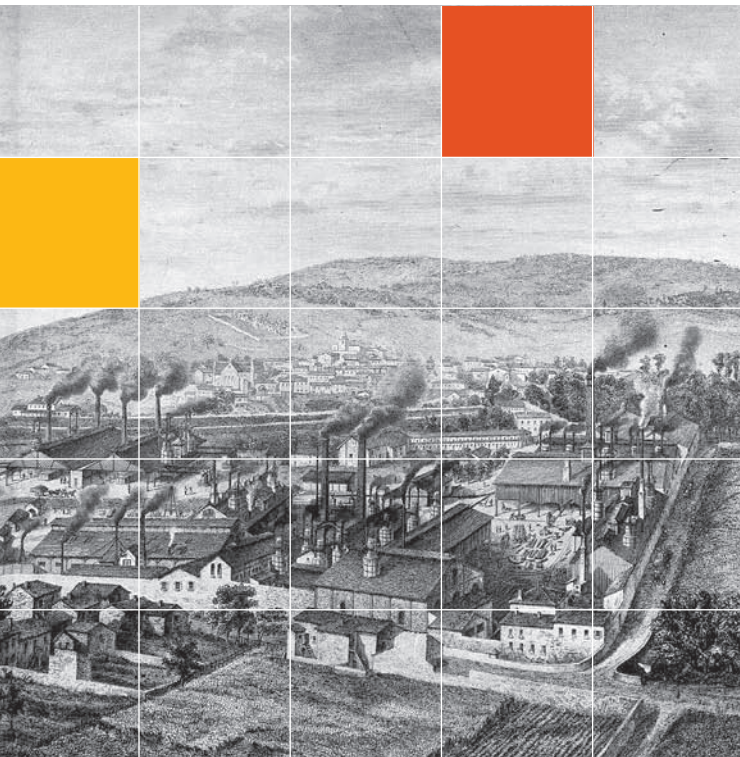
An installation of blast furnaces at the end of the 18 th century.
